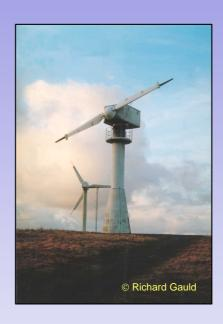
The 3MW and 250kW prototype wind turbines were designed and constructed by the Wind Energy Group during the 1980s. At the same time Howden completed their research and development of their 300kW wind turbine, with all three machines tested on Burgar Hill during the late 1980s and early 1990s. Although each design of machine functioned, and the site produced over 10GWh of electricity, design failings ultimately led to the demolition of these experimental turbines.
